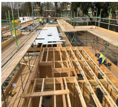
1. Engineered Metal Web Joists.
