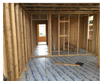
3. External Load-Bearing Wall Panels.
